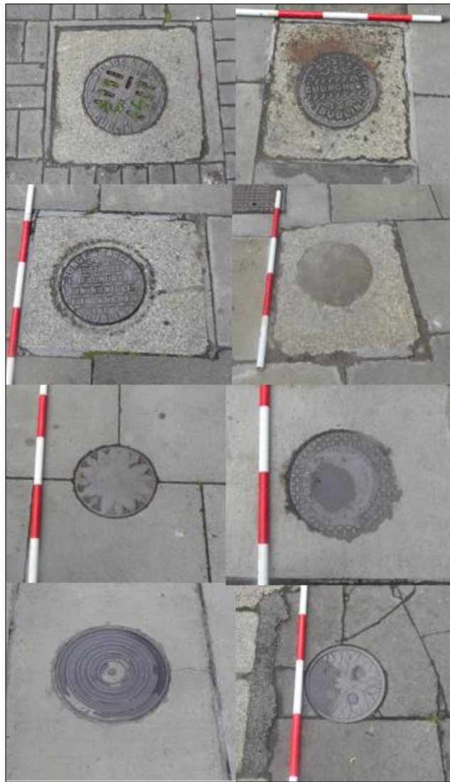
Sample of Coal Holes, covers and granite surrounds
